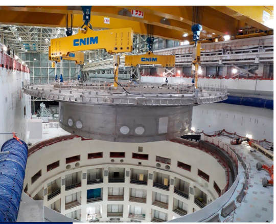
Handling the heaviest ITER component, the cryostat base weighing 1250 tonnes.
