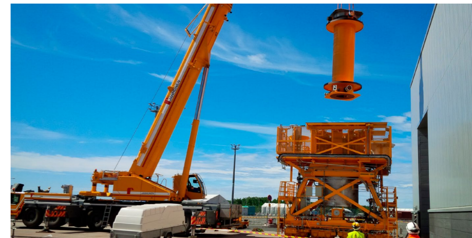
Load testing of the OL3 EPR's spent fuel cask handling trolley
